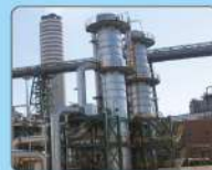
FLUE GAS DESULFURIZATION
